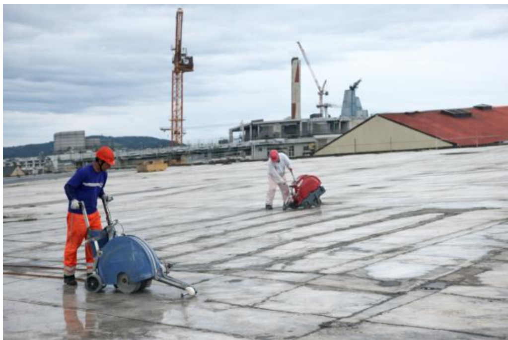
Figure 3: Cutting phase of the ribbed concrete slabs during the dismantling process, aimed at adapting the elements for reuse. Graphic by Parabase. © Parabase, with permission for publication.
