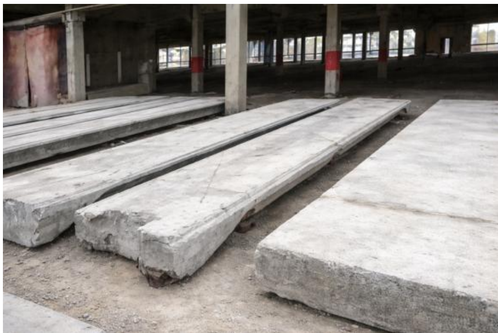
Figure 4: Failed outcome of the dismantling phase due to the use of a water-based cutting system, which caused excessive inaccuracies and prevented the reuse of the components. Graphic by Parabase. © Parabase, with permission for publication.
