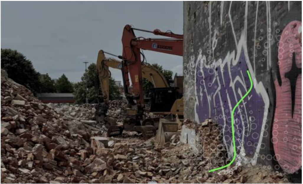
Figure 1: Photo of a demolition site on Bahrenfelderstraße in Altona, Hamburg. Project image by the Author, 2026
