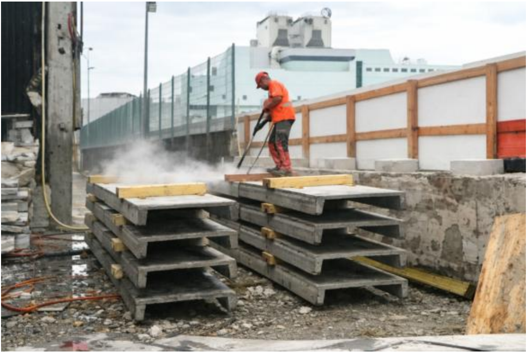
Figure 5: Cleaning phase following the dismantling of the ribbed concrete slabs prior to their potential reuse. Graphic by Parabase. © Parabase, with permission for publication.
