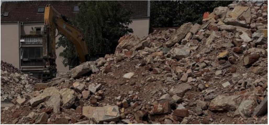
Figure 2: Photo from a demolition site in Hamburg. Everyday dissolution of brick architectures into undifferentiated rubble. Photo by Author, 2026.
