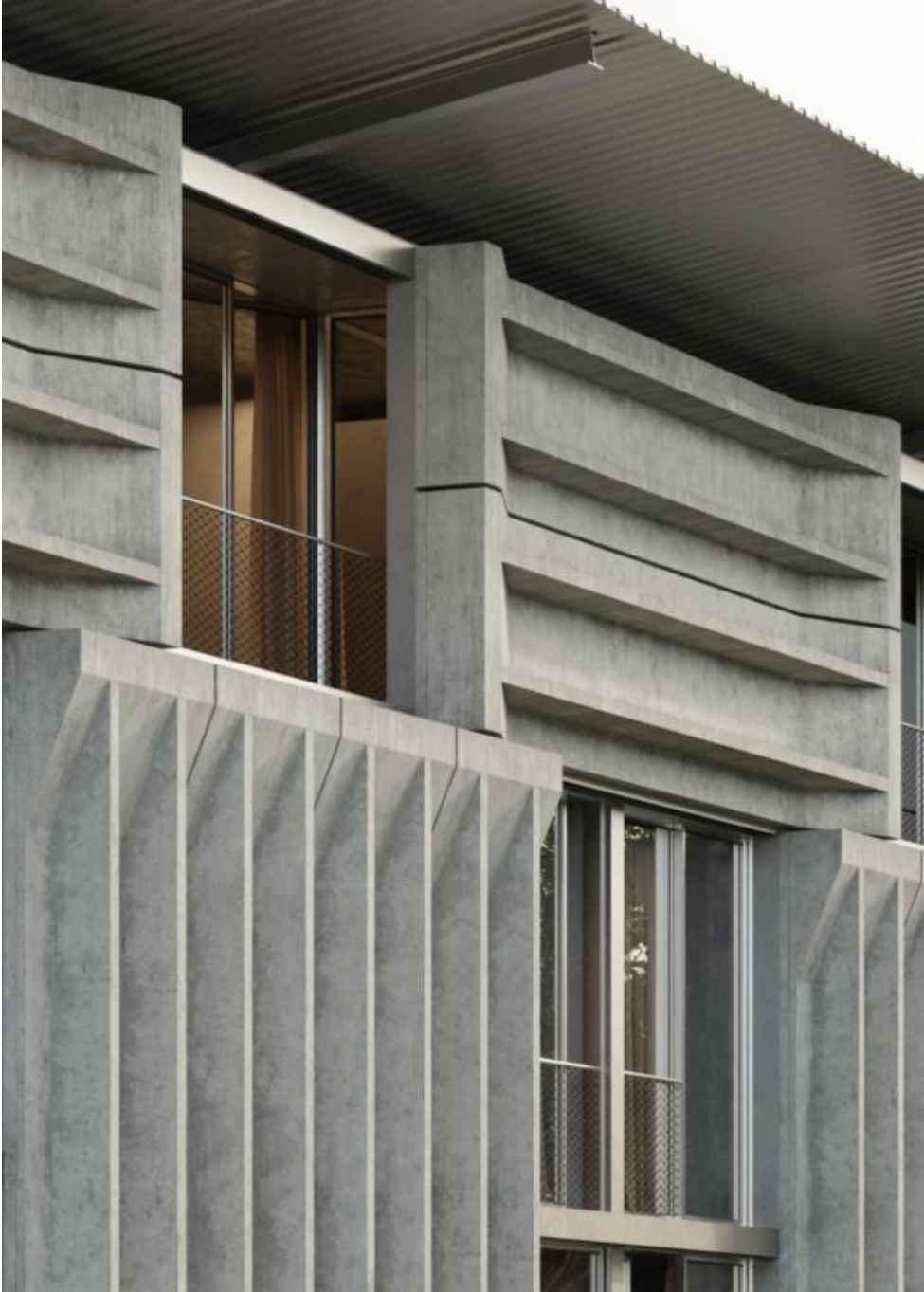
Figure 2: Detail view of the façade composed of load-bearing ribbed slabs reused from the demolition of the Lysbüchel parking garage. Graphic by Parabase. © Parabase, with permission for publication.
